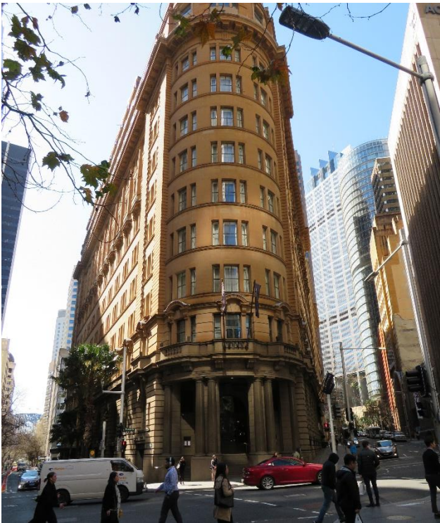
Figure 39 View east along Hunter Street, towards the heritage listed Former Wales House at the intersection
