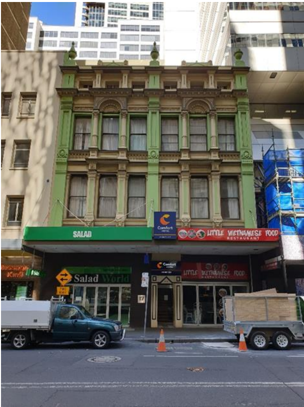
Figure 15 - Façade of 15-17 Hunter Street
