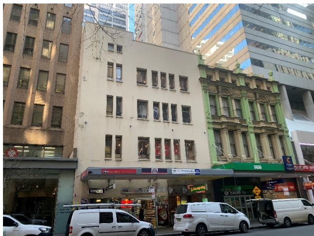
Figure 23 The principal northern Hunter Street façade
