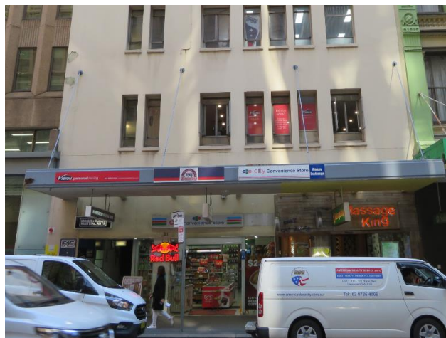
Figure 24 The ground floor shopfront
