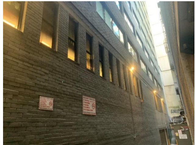
Figure 30 The northern Empire Lane façade
