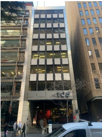
Figure 29 The principal Pitt Street façade
