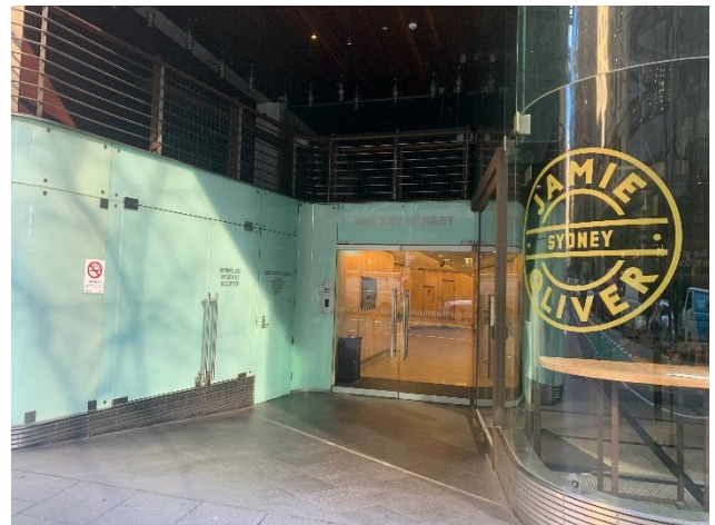
Figure 32 The ground floor lobby and restaurant entries
